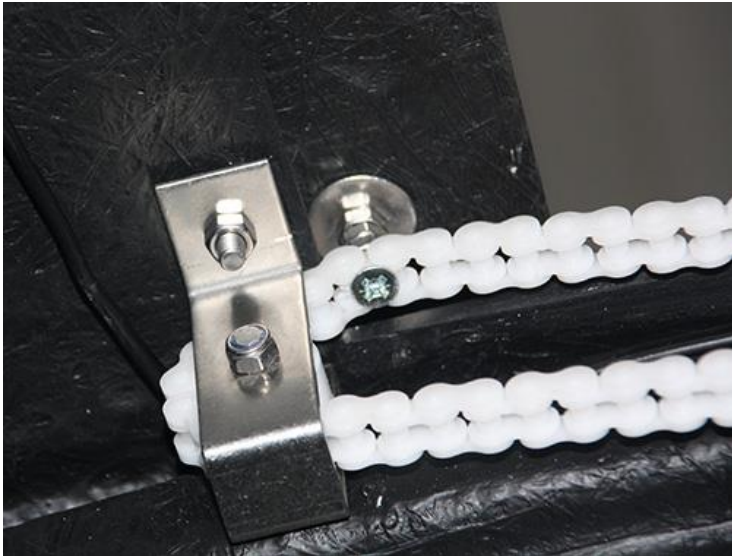
Rear bracket shown with shutter fully open
